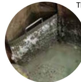
The mesh of the screening should be smaller than the smallest pellet handled at the facility.
